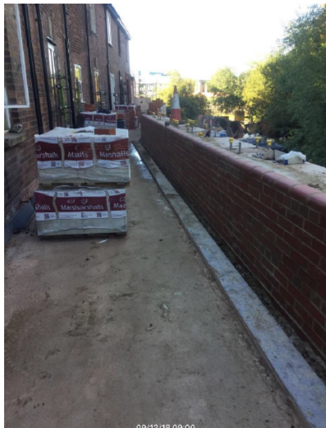
Work on balcony wall at Eagle Cottages, upstream of The Mill on the Exe, prior to installation of glazed flood barrier.
